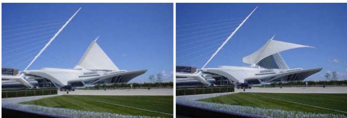
Figure 3.8 Milwaukee Art Museum Roof Structure Open and Close Movement [7]
