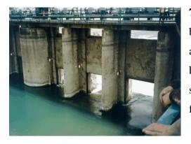
**7.12** A gated diversion weir has b=3m net gap between ten gates. When the gates are open at a=1.6m, the downstream water level of the weir is h=5.8m at the stilling basin. Determine the submerged flow conditions, calculate the total flowrate under the Gates.
